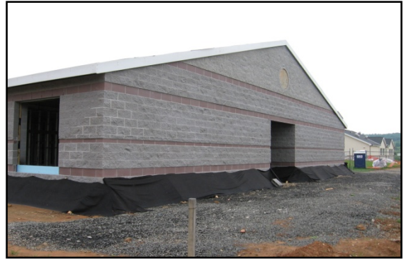
Exterior of Upper School Humanities & Instructional Technology Wing.
