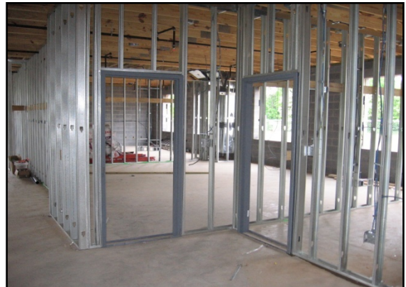
Interior of Upper School wing takes shape and classrooms take form.
