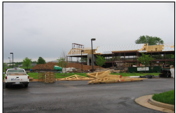
Trusses installed on new Lower School.
