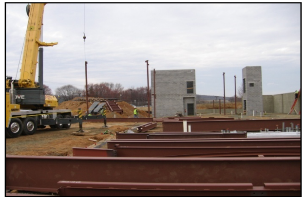
Steel being put in place at Lower School
