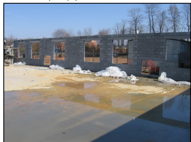
Exterior Wall for the Upper School Humanities & Instructional Technology Wing
