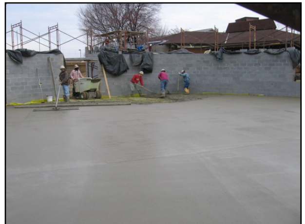
Rotunda walls partially up and slab finished.
