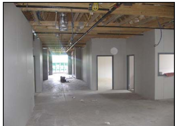
Upper School Rooms – Drywall is installed
