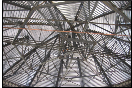
Rotunda Ceiling – Metal Trusses and Piping
