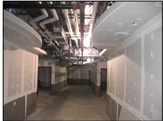
Bulkheads at Corridor in East Wing
