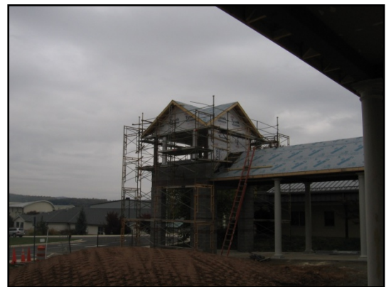
Breezeway copula with columns in place
