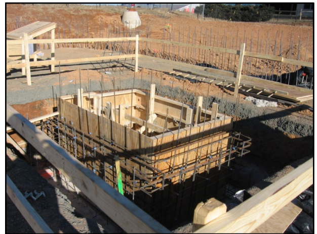
Construction of the elevator pit
