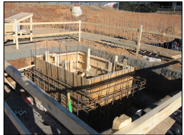
Construction of the elevator pit
