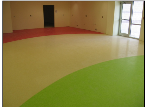
Installation of VCT throughout
