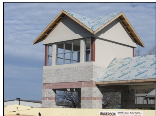
Metal Roof on Cupola
