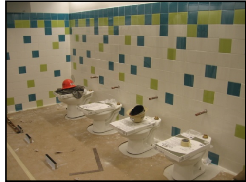
Installing fixtures and toilet partitions
