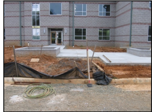
New Sidewalk and Planters
